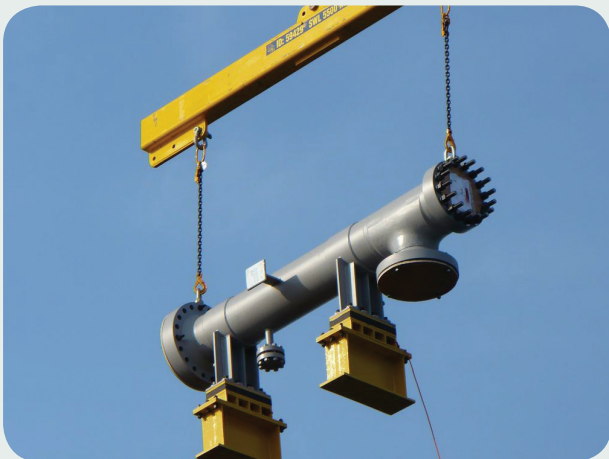
Installation of Production Boosting Ejector for Shell, Southern North Sea
